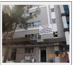
NC-4: The main entry door, that has been identified as emergency exit gate is a shutter gate, does not open outwards which does not comply with the local regulations.
