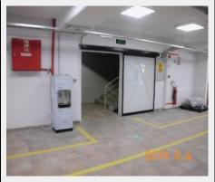
NC-6: The production sections in each floor have emergency exit gates that are sliding glass doors, which does not comply with the local law.
